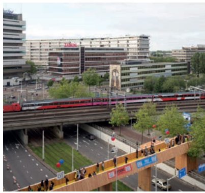
Temporary infrastructure Luchstingel bridge, NL
